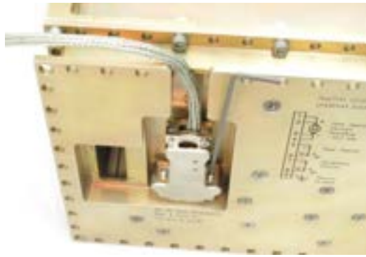
Figure 20-4: Installing CSD initiator electrical harness
